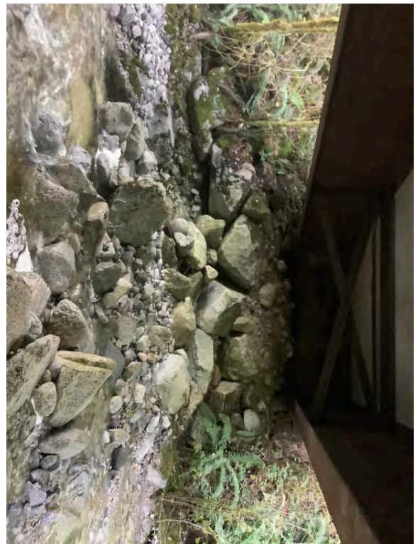
Right Bank Abutment when facing downstream
