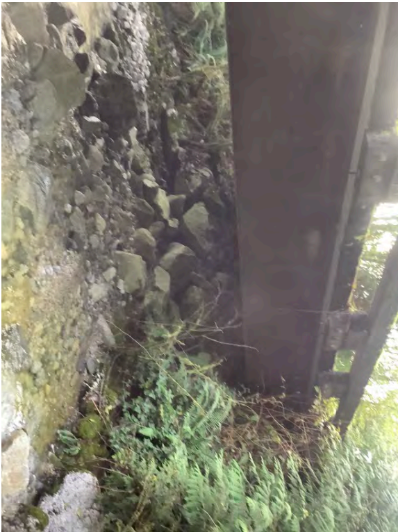
Right Bank Abutment when facing downstream
